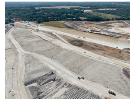
2 Chalk excavated for HS2, laid out near the south portal of the Chiltern Tunnel, 2022
